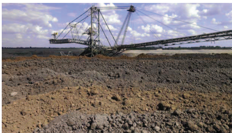
Picture 11.1 Backfilling of an open-pit mine.
