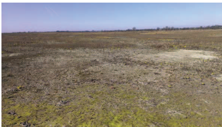
Picture 11.3 Areas before starting the remediation process.
